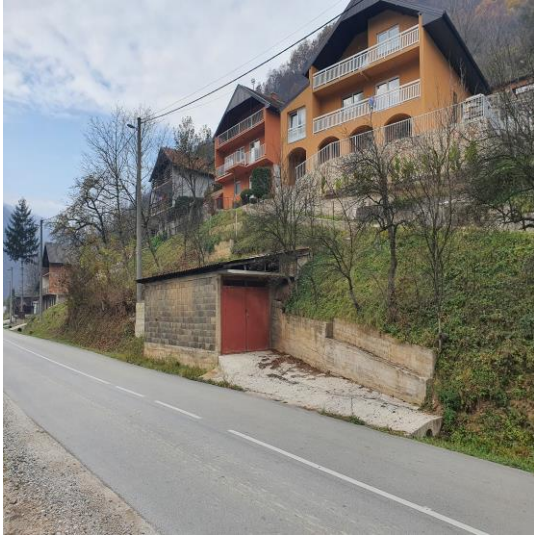
Figure 7 – Garage in Janjići settlement
