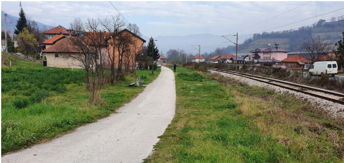
Figure 12 – Belt between the existing railway and the existing local road where the transmission pipeline should pass in the settlement of Janjići
