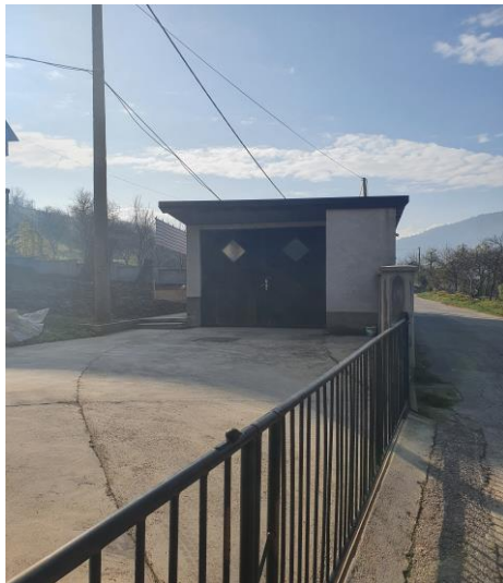
Figure 9 – Garage in Putovići settlement
